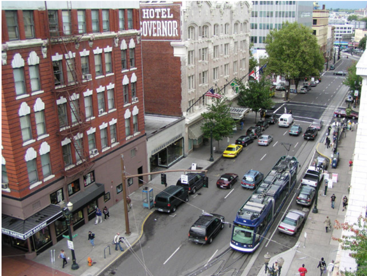
Rail Placement in Second Lane in Portland, Oregon Transit System (Photo courtesy of John Smatlak, Railway Preservation Resources, from www.railwaypreservation.com )
